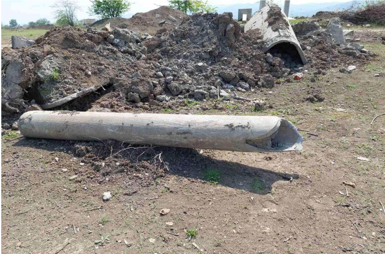
Asbestos pipe at the construction site
